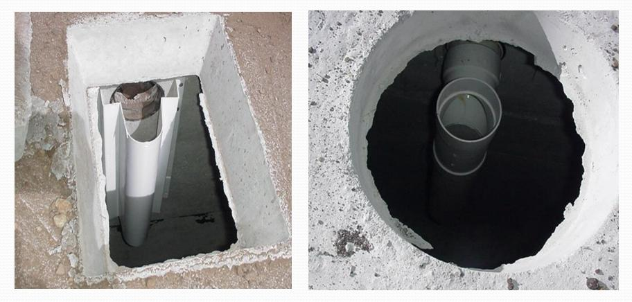
Baffles help protect the drain field, by keeping solids in the tank
