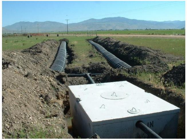
Effluent from the septic tank is directed equally into each drainfield leg
